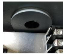
3 b) – Feed wires through hole into fixture
